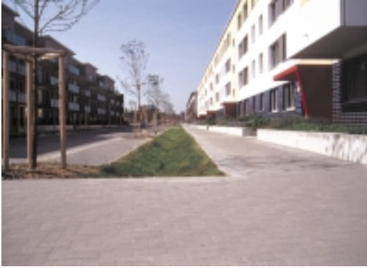
Street-laid gully and trench system
