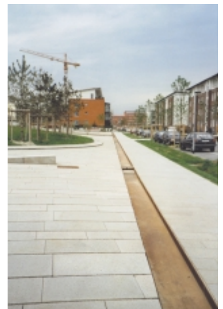
Boxed-in drain with sound opening
