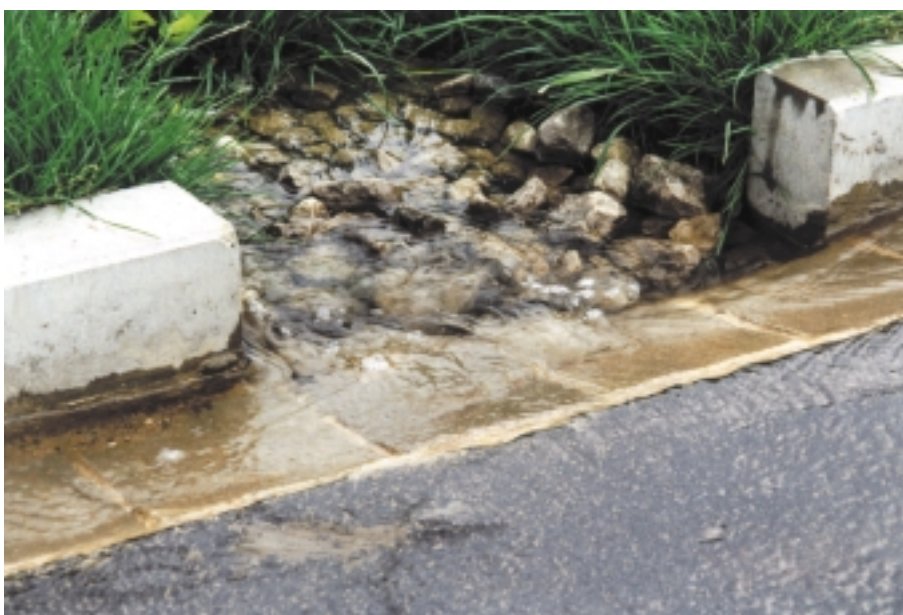
Gulley lead with ballast packing
