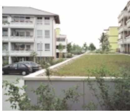
Carport with roof planting
