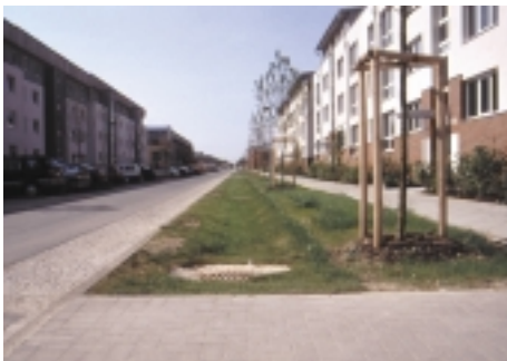
Gulleys at Ellernbuschfeld
