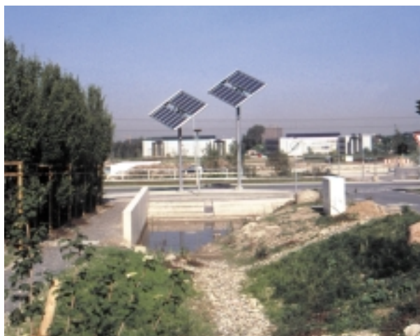
Photo-voltaic plant on the slope of Weinkampswende
