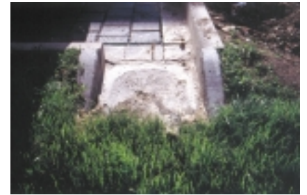
The new gulley inlet
