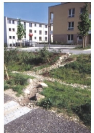
Weinkampswende - rainwater channel
